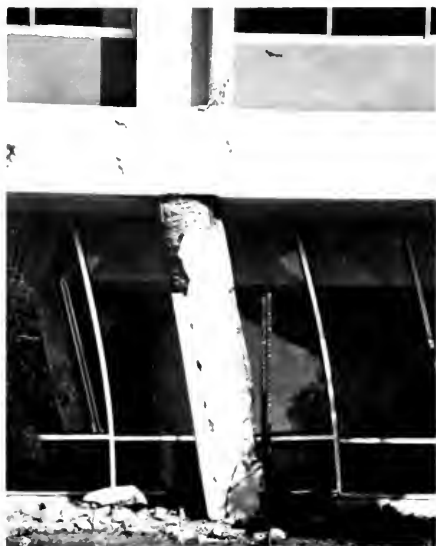
Photo 24. Spirally wrapped reinforced concrete column; compare with tied column (photo 25). Note distorted mullions for glass and about 2-foot offset in first story.
